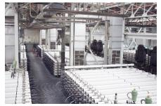
successful 30 MGD RO expansion in 2015 as an example of a community using wastewater reuse as a creative solution for preserving groundwater reserves and protecting aquifers from seawater intrusion. The OCWD Groundwater Replenishment System (GWRS) relies on RO membrane technology to replenish natural freshwater barriers to saltwater intrusion and to provide much needed aquifer recharge with secondary treated effluent from local municipalities. Today, at full operation, the OCWD
